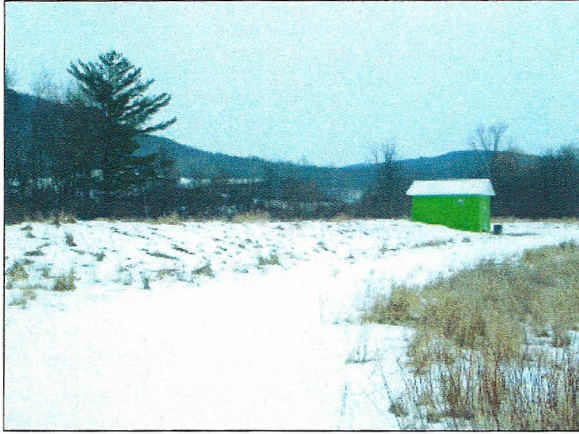
Figure 3. Well Point Field and Pump House
