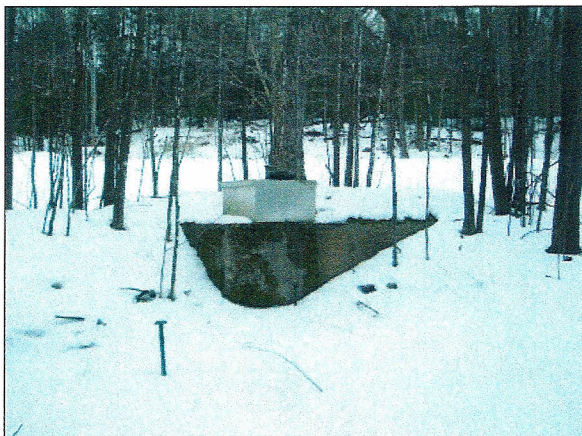
Figure 5. Maple Ridge Cistern
